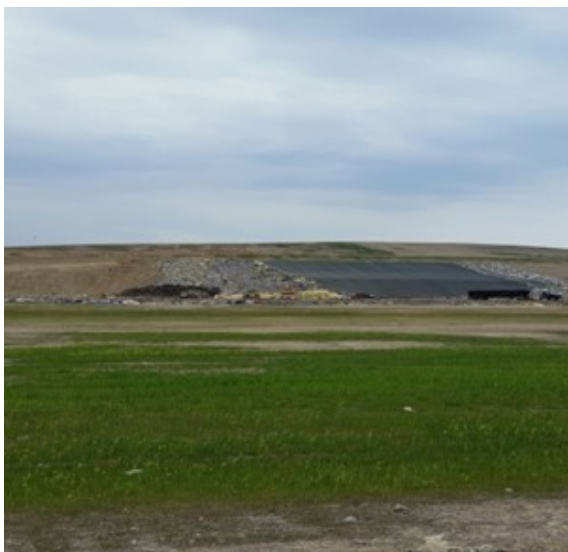
Placing Select Waste
