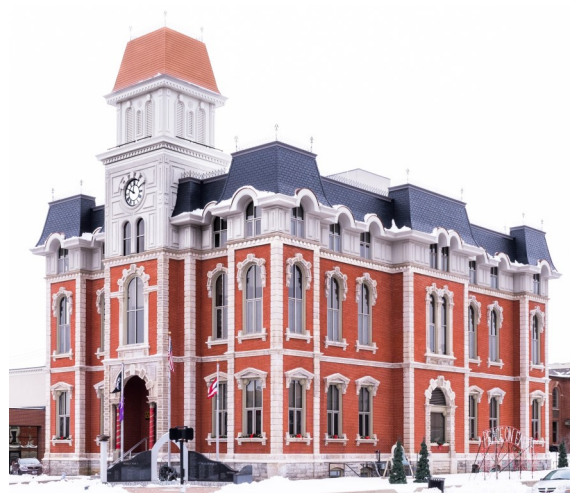
After 2016 Renovation Project
