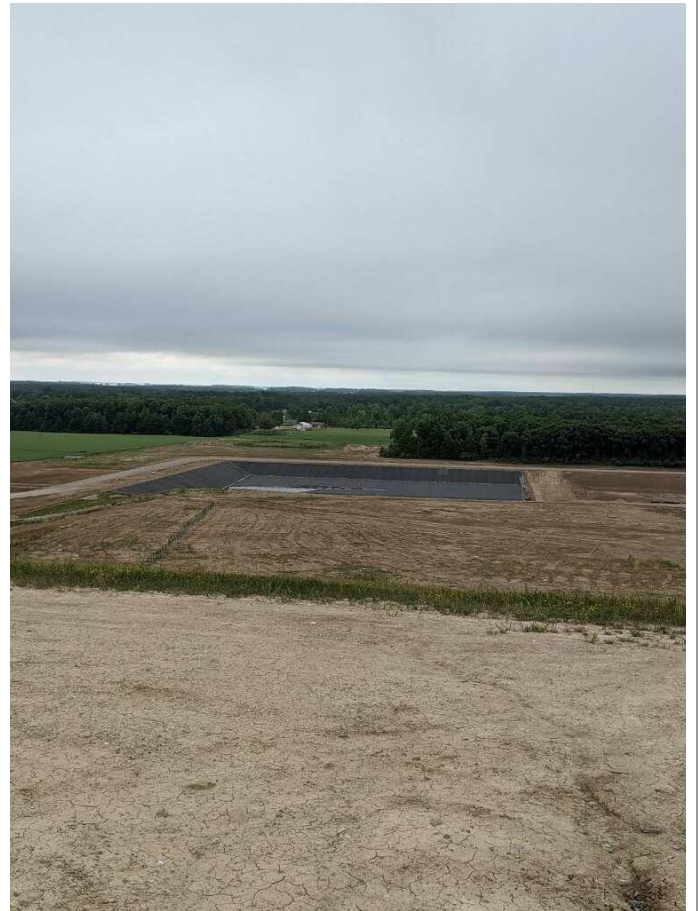
View from the top of the existing Landfill looking southeast towards Cell 5
