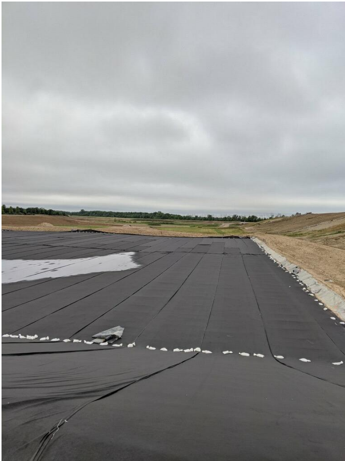
View of the new liner from the east.
